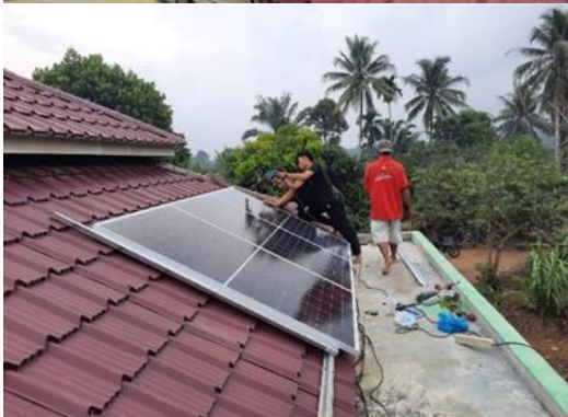
Gambar 7. Pemasangan Panel Surya Di Rooftop Masjid Ar Rohim
