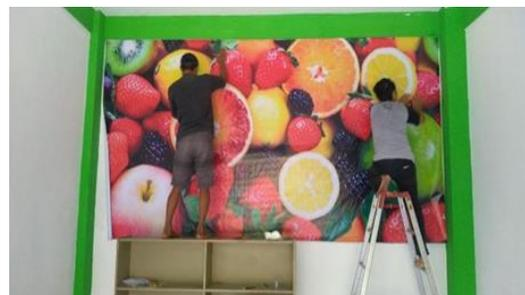
**Gambar 7. Proses Pemasangan Wallpaper Dinding Bagian Dalam**
